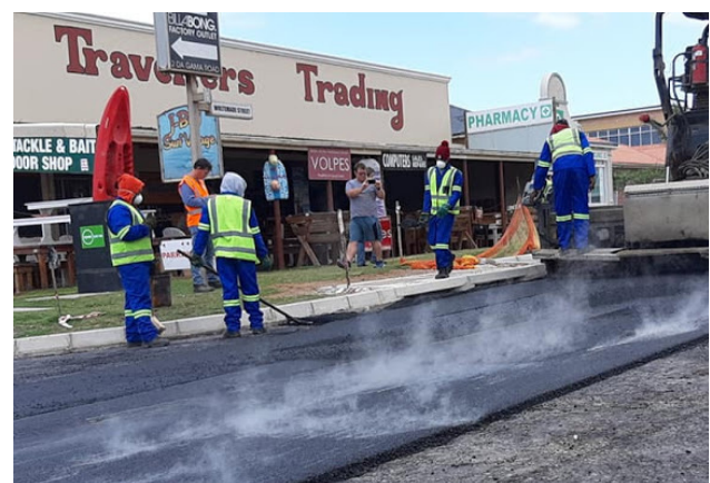
A street in Jeffreys Bay is repaired by making use of plastic waste.
