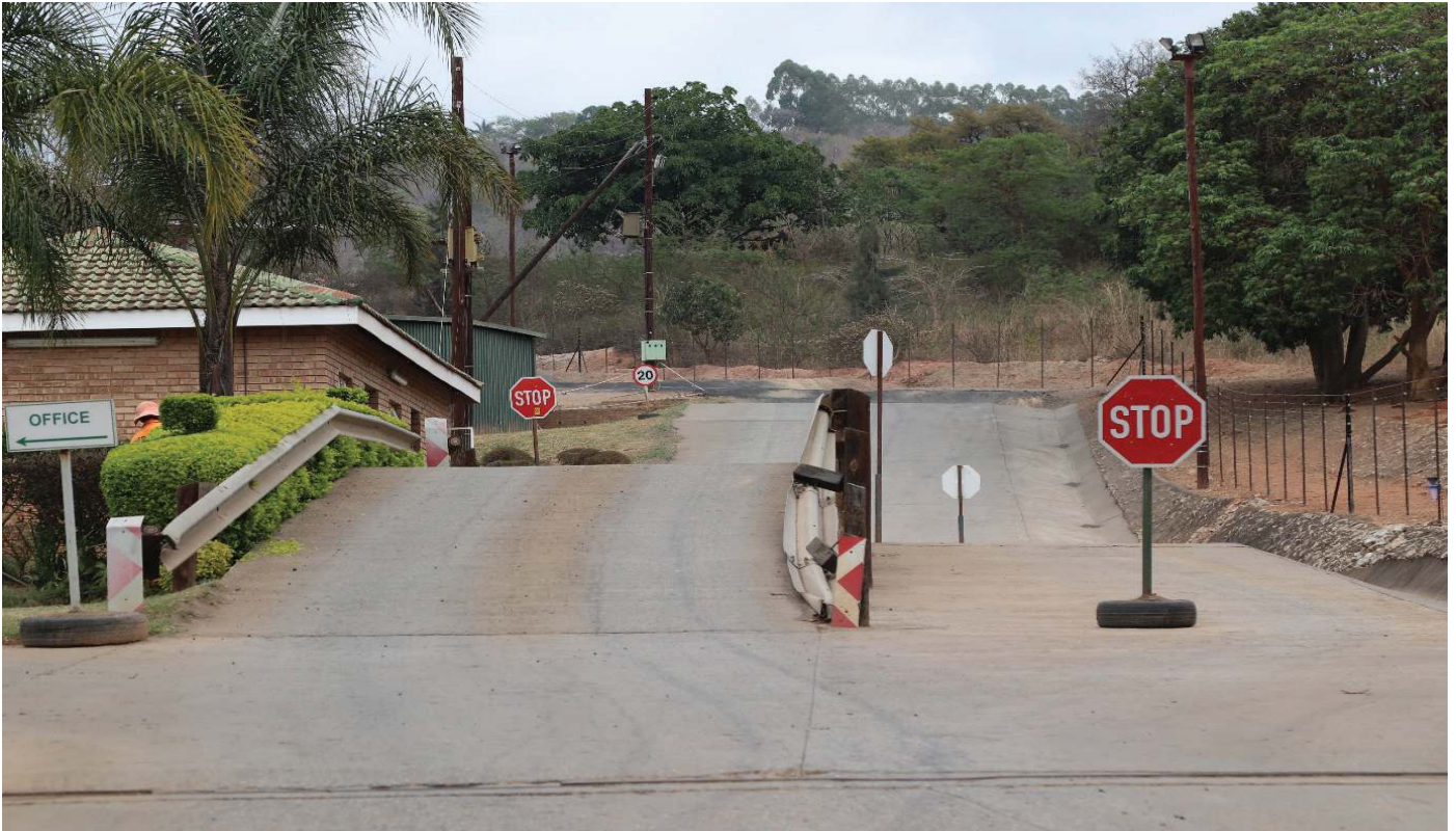
An impeccable landfill site in Tzaneen, with an operative weighbridge, fence and complete infrastructure
